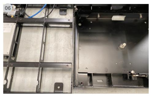
11. Fix the sensor housings to the floor, use four fixings for each housing.
